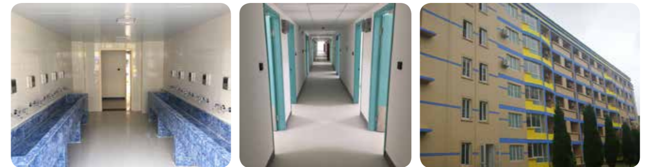
Employee dormitory renovation
