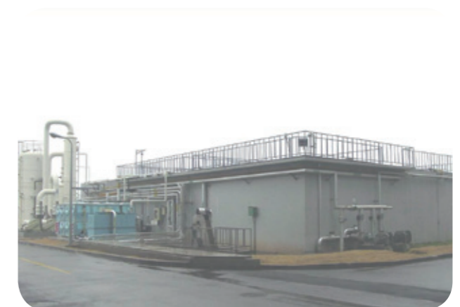
Domestic Sewage Treatment Facility
